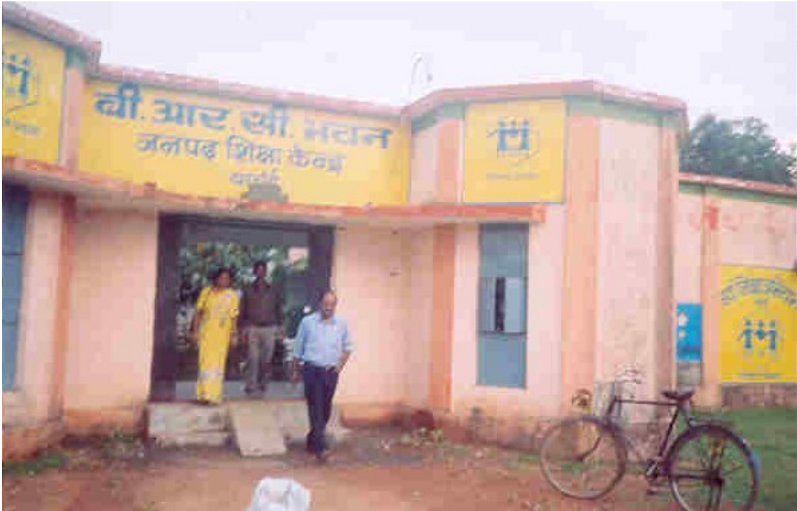
Plate 15: Block Resource Centre (BRC), Bawai block, Hoshangabad
