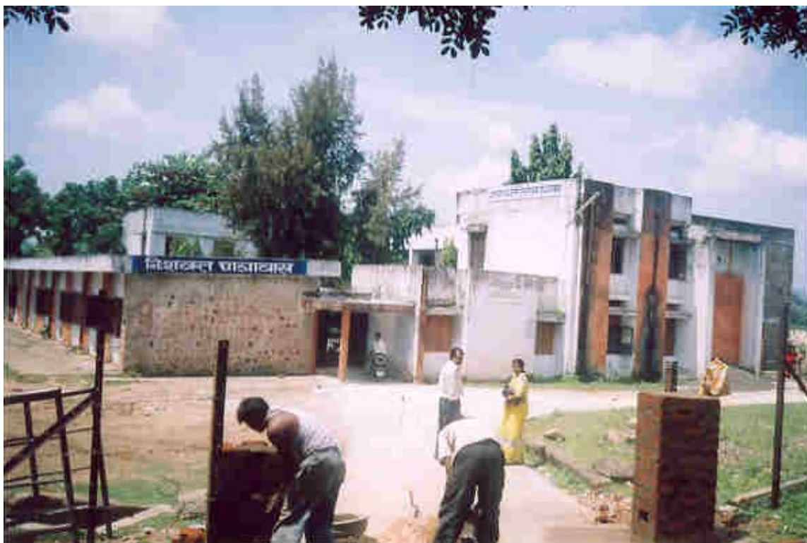
Plate 7: Hostel for Children With Special Needs
