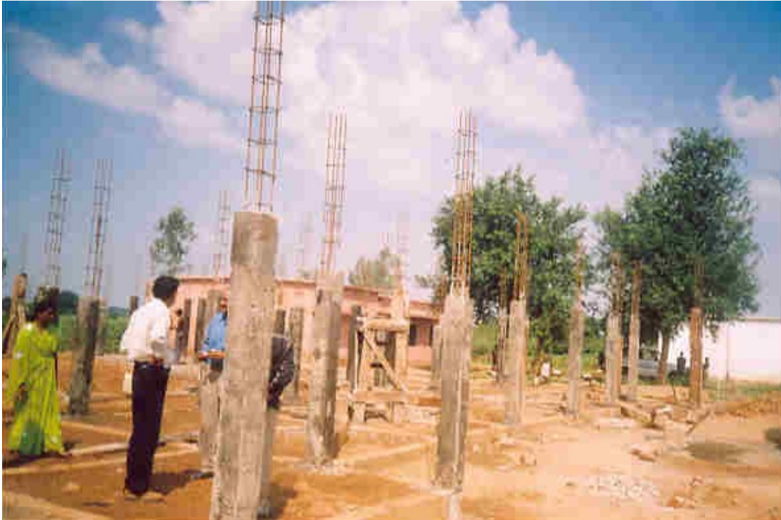
Plate 4 : A KGBV hostel under construction
