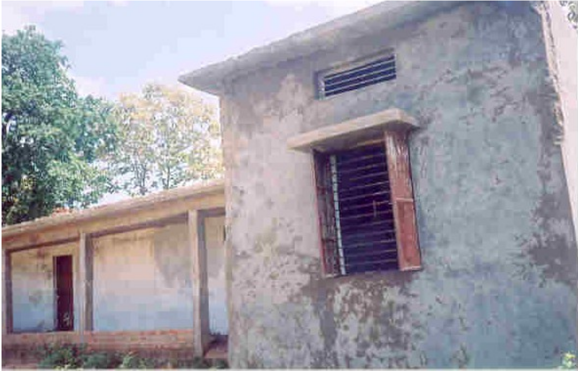
Plate 3: Completed building for a Middle school
